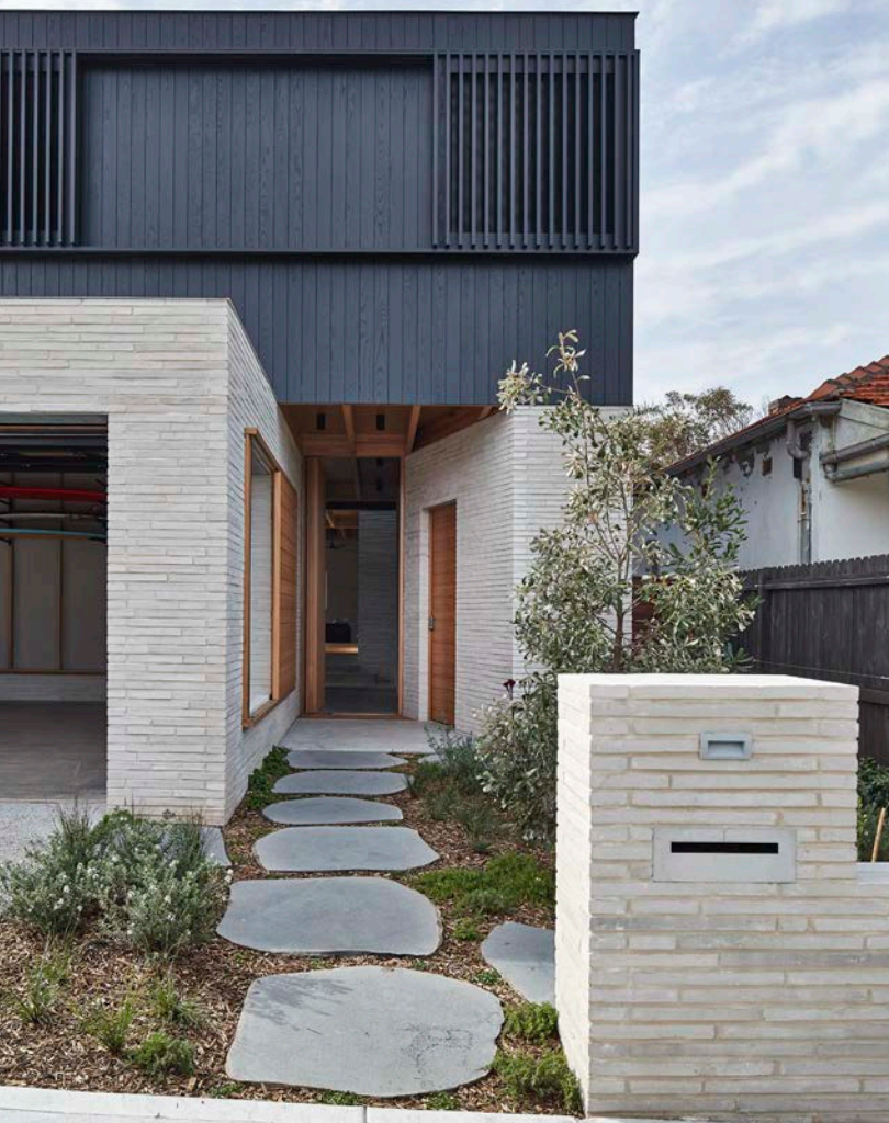
02 From the street, the new house presents as stacked cubic forms.
